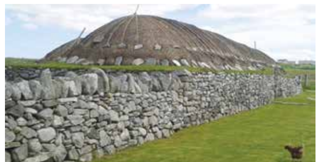
Fig 2- The Arnol Blackhouse, Isle of Lewis, Scotland. The walls are constructed as inner and outer dry stone skins, with the largest stones at their base and smallest at the top, and the core infilled with compacted earth. This solid construction, up to 2.1 metres thick, provides excellent protection as well as insulation against often severe weather conditions allied to singular comfort conditions. Source of image: author
