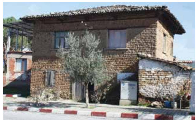
Fig 1 - Load bearing adobe: house in the town of Konaklı (Adagüme) near Tire, Izmir Province, Turkey.
