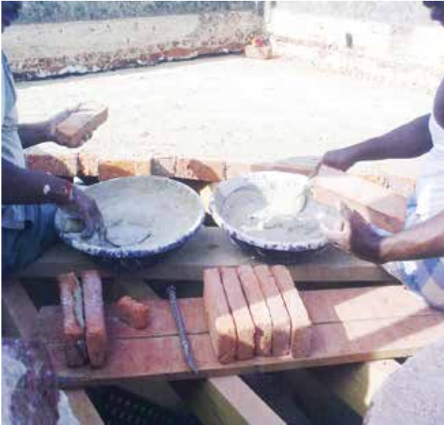
4. Laying of the Madras Terrace with bricks made in the local kiln.
