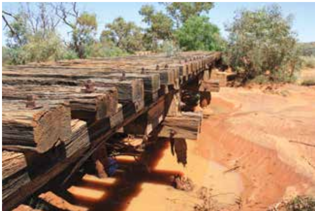
The heritage railway bridges on Rupee Station were constructed of giant timbers cut from River Red Gum, large specimens of which are now rare due to unsustainable harvesting
